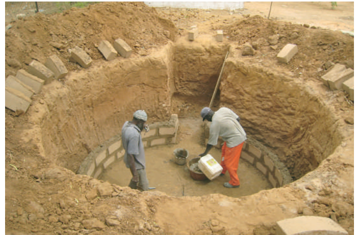
Masons from the community of Ouarkhokh are working with CREATE! to build a biodigester that will provide methane gas for lighting and cooking.
