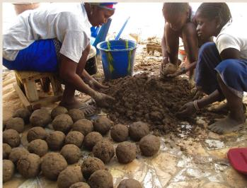
Next, the participants mix the ingredients together using their hands and feet until the materials are well combined. Then, participants should form the material into fist-sized balls. To confirm that the mixture is the correct consistency, drop a ball from shoulder height. The dropped ball should maintain its round shape, but be flattened on one side.
