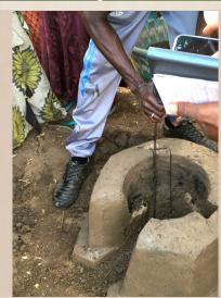
Next, participants cut two chimneys into the inside of the stove. These chimneys should be cut between the stones and should be two fingers deep. After cutting out the chimneys, participants can also use water to smooth the stove's inside walls.
