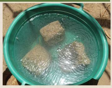
Participants should wet the bricks or stones with water. The bricks or stones should be of equal height so that the pot rests evenly on top of them. Participants can cut the bricks with a machete into equal sizes, if needed. Alternately, participants can dig a small hole for one or more of the stones to ensure that they are of equal height.
