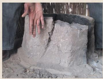
In the future, participants can repair a cracked cookstove. First, they make additional cookstove building material. Then, an individual uses their machete to smooth out the sides of the crack and moistens it with water, before using the cookstove building material to fill in the crack. Finally, participants should let the stove dry completely before use.
