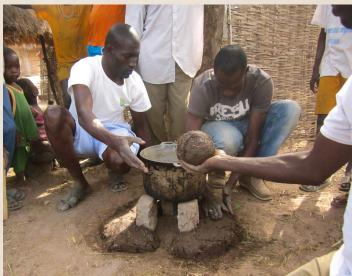
Participants then begin to build the cookstove. The walls should stay within the cookstove pattern. Walls should be a handswidth thick around the cookstove and walls should be straight from top to bottom.
