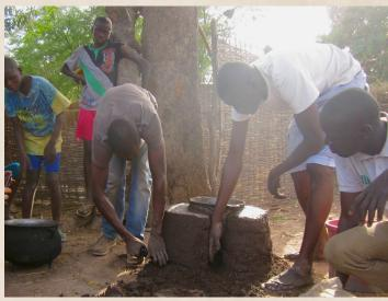
When building the cookstove walls, participants should construct an entrance to insert firewood. For small and medium cookstoves, this entrance should be the width of a fist with the thumb outstretched. For large cookstoves, this entrance should be the width of a fist with the thumb and pinky finger outstretched.
